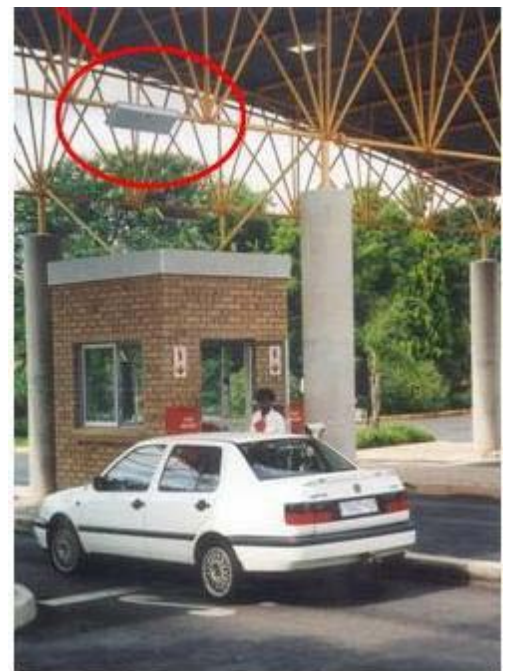
RFID controlled entrance – Reader circled
