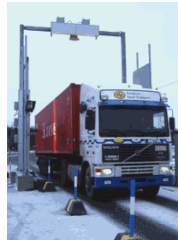
Truck and Trailer pass through the RFID entry/exit portal
