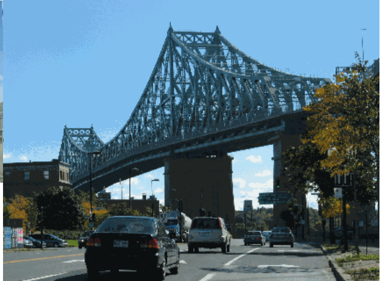
Main Cantilever Span of the Jacques-Cartier Bridge
