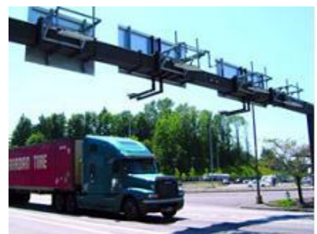
A transponder mounted in the cab of the truck relays information to the roadside electronic reader through antennae in the overhead structure. Source: FHWA
